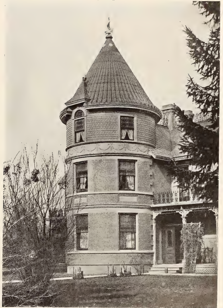
No. 690—Illustrates circular tower of a Chatham, Ont., residence, roof of which is finished with our graduated tiles.
